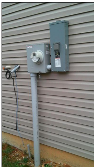
Main Electrical Shutoff.
